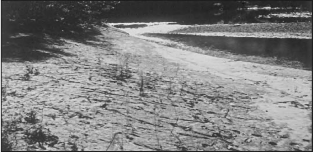
Figure 6.37 Willows and other live stakes will root and sprout rapidly to protect slopes. The roots form an interlocking mat to hold soil in place, while the foliage protects the soil surface. These willows, planted along Hinkson Creek in Columbia, were 3- to 5-foot tall within six months. Source: Doug Wallace. NRCS. Boone Co.
